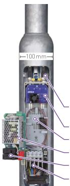
The ultra-compact junction box **PE-LIGHT** integrates power connection and passive or active unmanaged/managed data transmission into the fiber optic network in the light pole; it is the smart node for the future Internet of Things on corporate sites or in smart cities.
