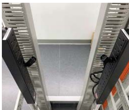
PDUs and cable management in the rack
