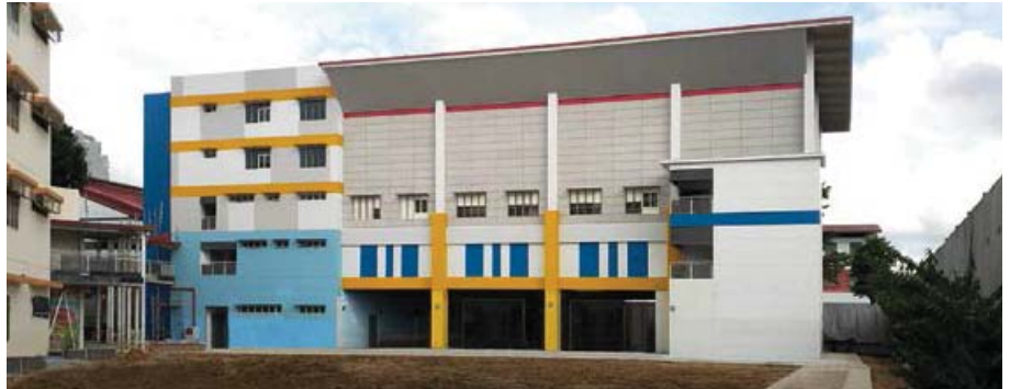
Zhenghua Primary School during construction
