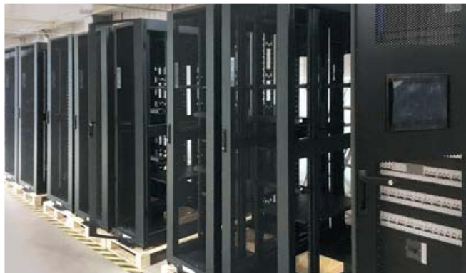
On-site installation of the IT infrastructure at the Ctrip site in the Philippines
