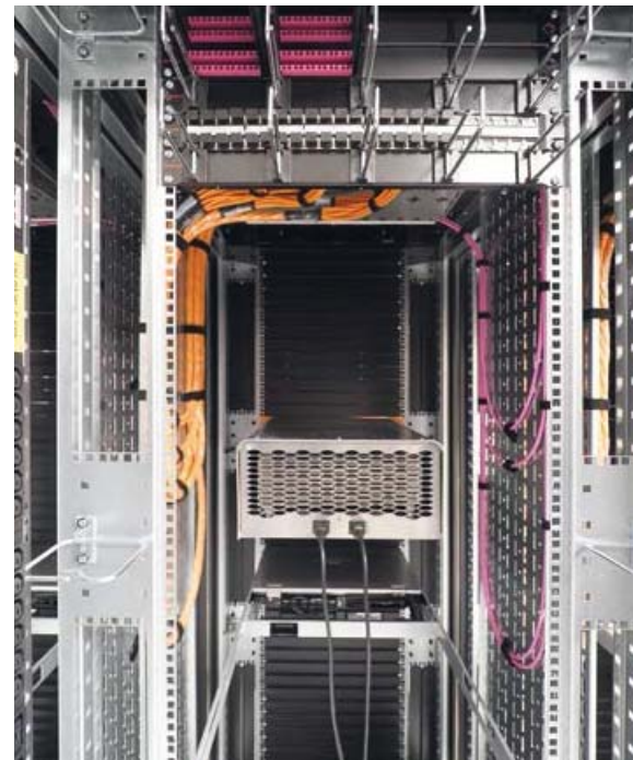
A look from the rear: server rack during the acceptance test
