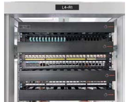
Copper, fibre and cable management panel installation
