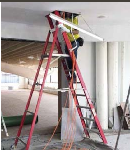
Installer pulling cables through the ceiling
