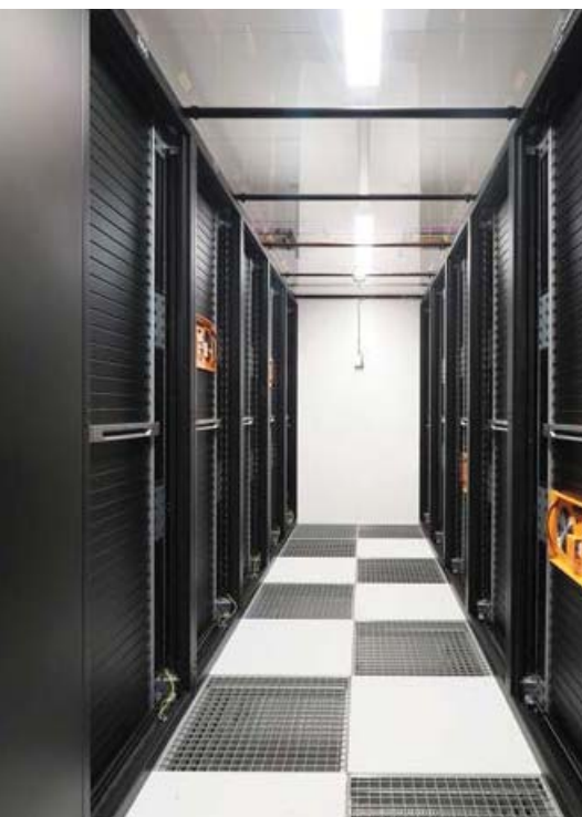
Server rack containment with load banks during the integral test
