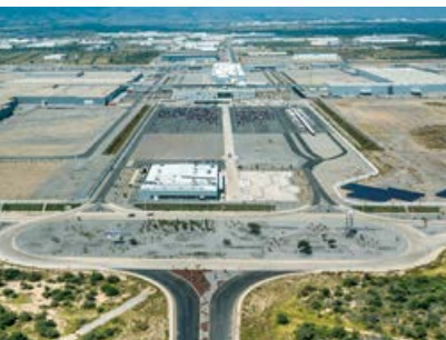
Car manufacturing plant, equipped for the future – page 8
