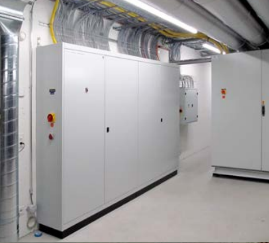
Plant room installations
