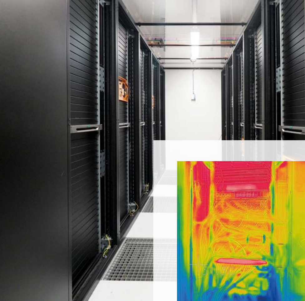
Image left: Thermoscan of a rack in a Datwyler customer's data centre
