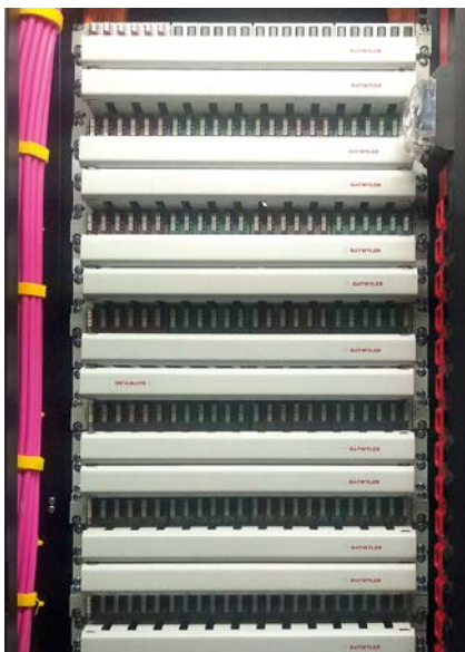
Rack in the YTO data centre
