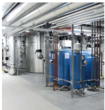
View in one of the plant rooms
