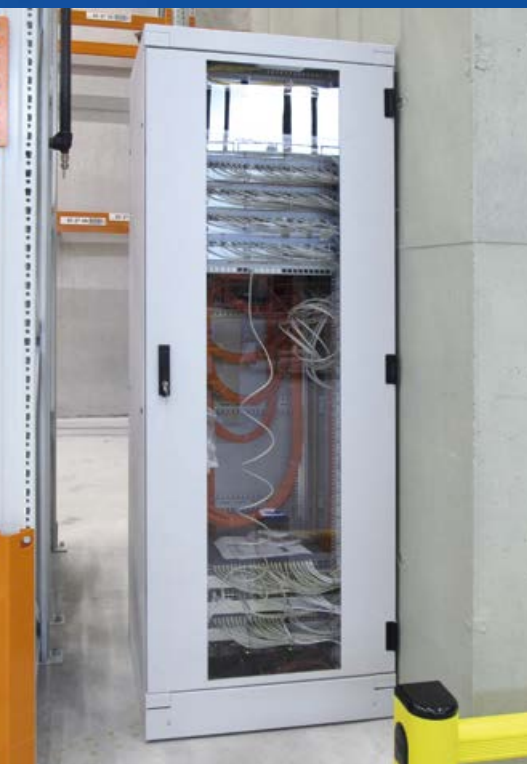
IT rack on the ground floor
