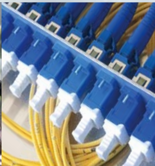
The mobile fibre optic closure
