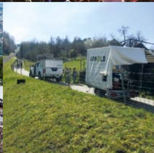
Installing the cable along the Gurtenbahn railway line
