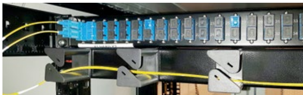
Photo right: fibre optic patch panel
