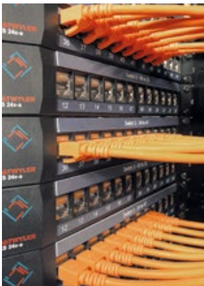
Picture left: angled copper patch panels in the network rack
