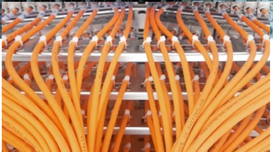
Photo right: Category 6 A cable and connection technology from Datwyler
