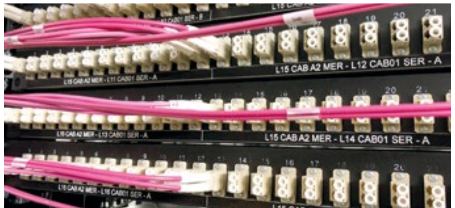
Fibre optic panels
