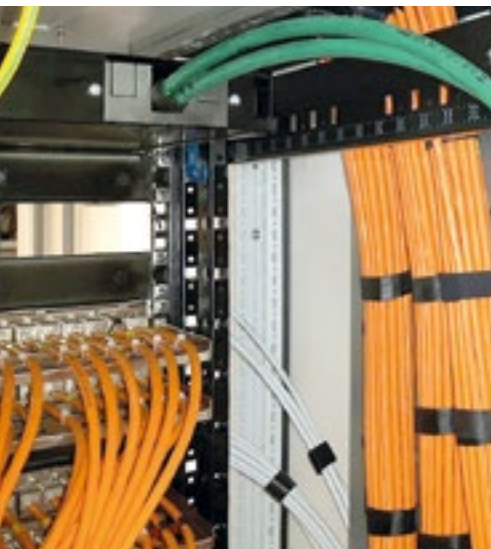
Neat cable management in the distribution rack
