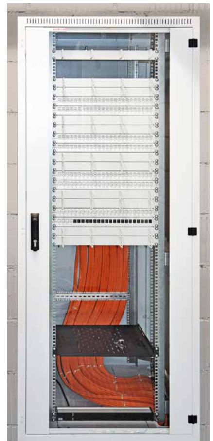
Looking into a network rack
