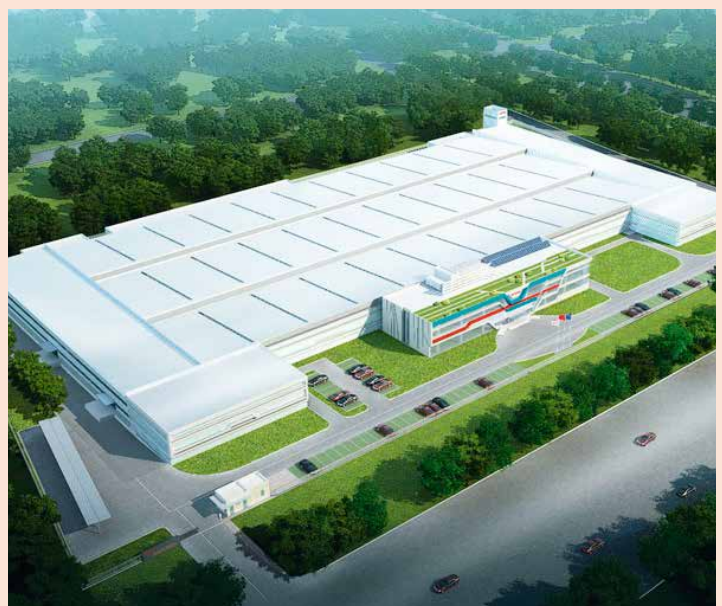
Datwyler (Suzhou) Cabling Solutions Co., Ltd. in Taicang
