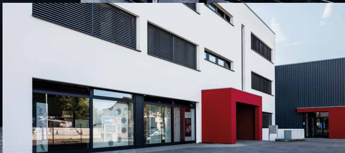
Main entrance to the new data centre and support centre
